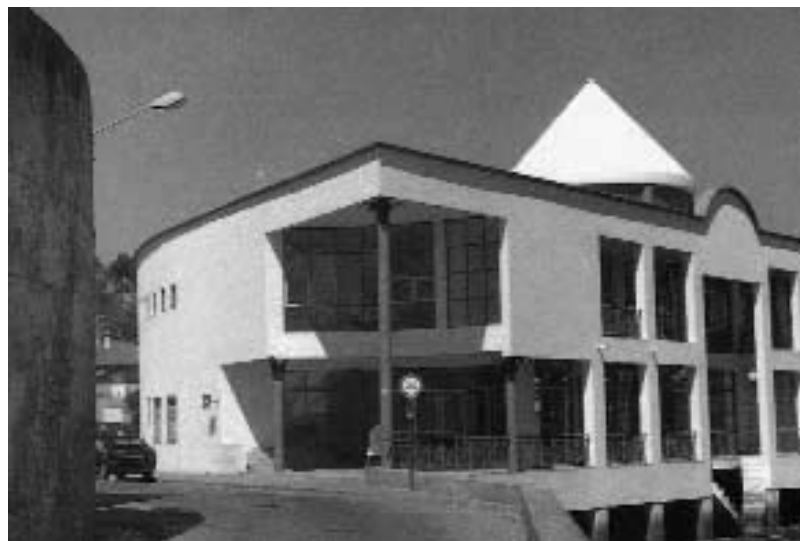
Figure 3.13 Bus Station, Tavira, Portugal
